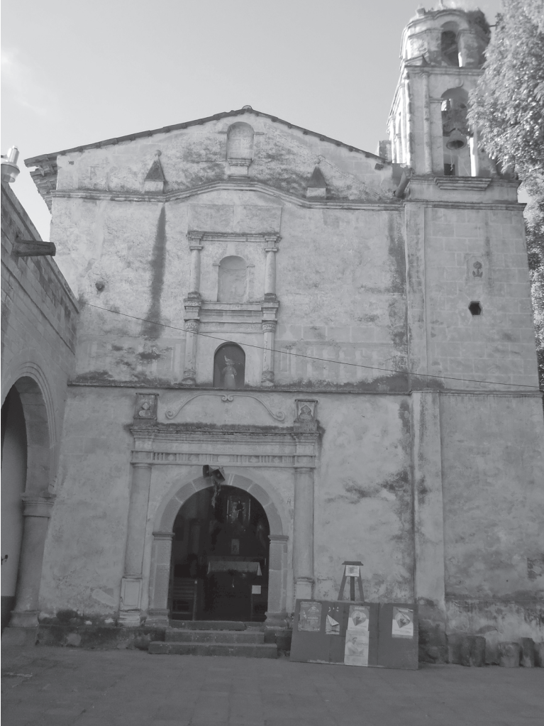
FIG. 5 Facade of the church of the Tercera Orden de San Francisco in Calimaya, the original church attached to the Franciscan convento. Photo: authors.
